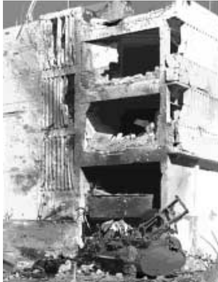
US Embassy Damaged by Terrorists in Tanzania
