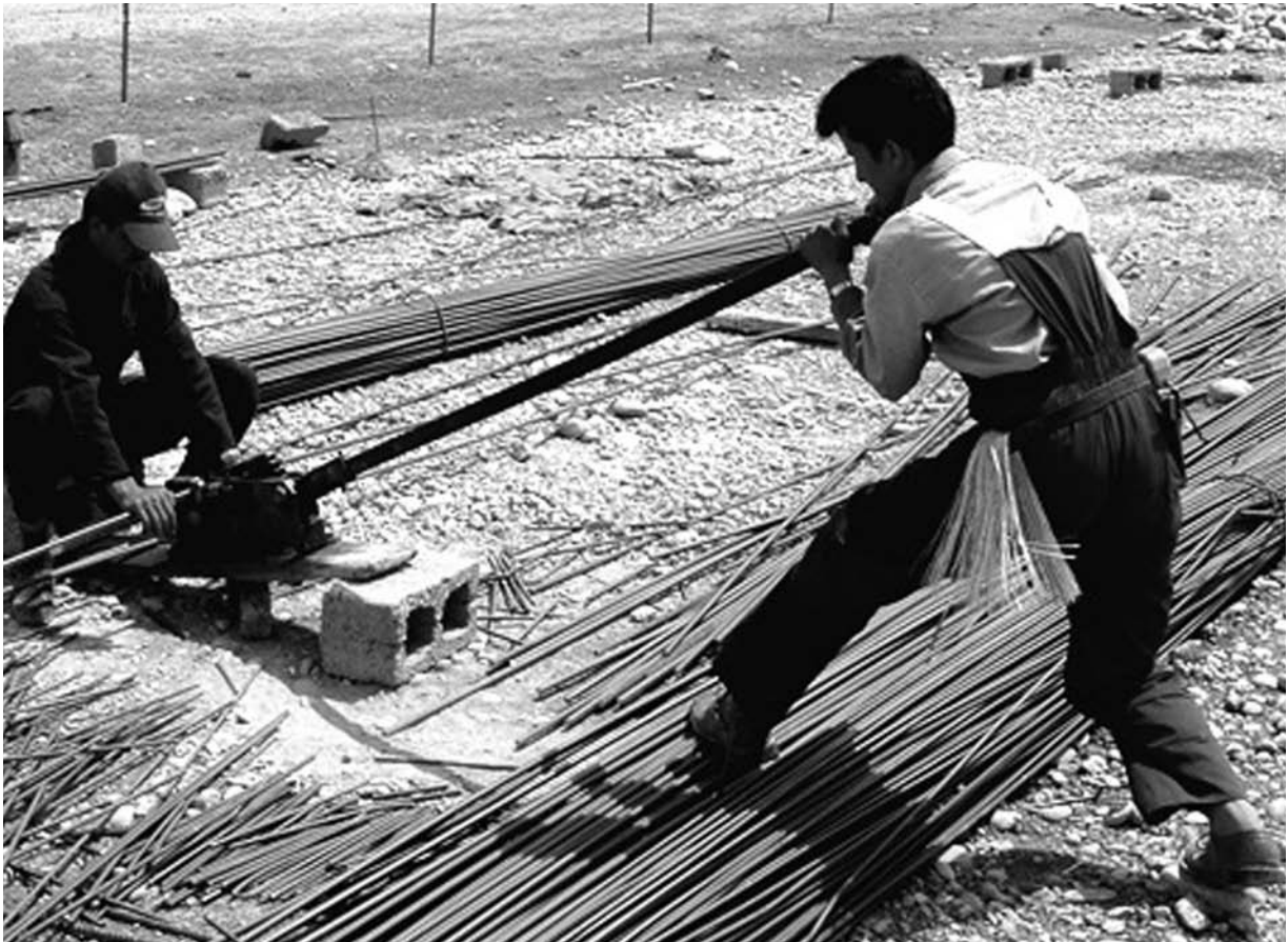
Iraqi subcontractors cut rebar for a health care clinic under construction outside of Erbil, Iraq, 20 June 2005. The clinic will handle primary health care requirements for a suburban neighborhood outside of Erbil. The U.S. Army Corps of Engineers oversees the project and works directly with Iraqi workers and contractor companies.
