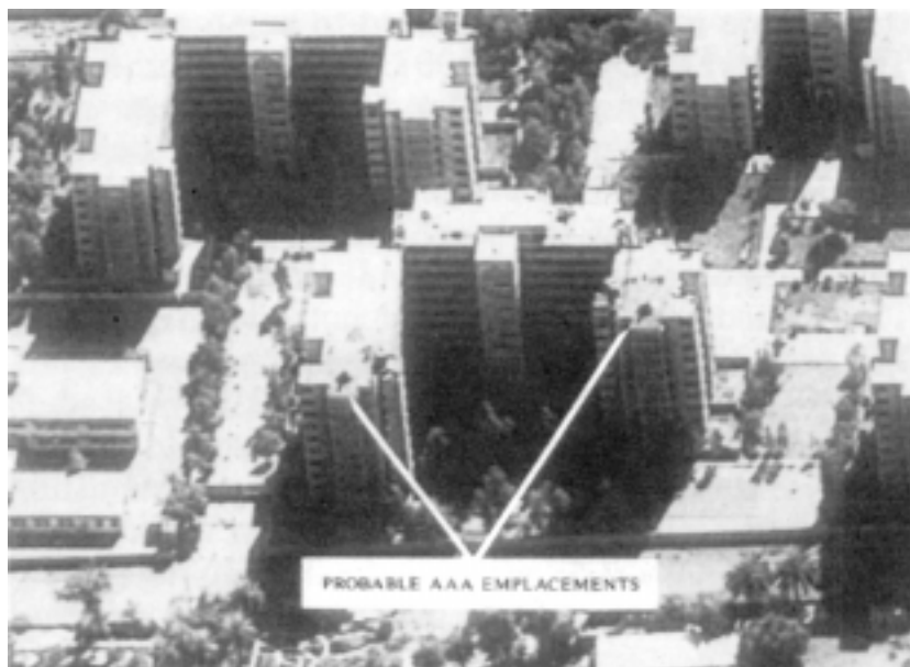
A pair of 5-mm anti-aircraft guns atop a civilian apartment building in Baghdad, 1991.
